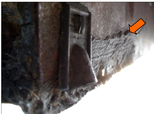
Trunk drop sealant Drain added later
