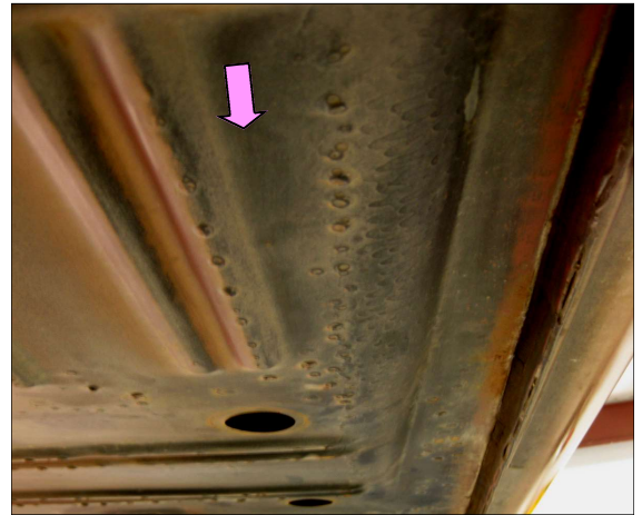
Floor behind rocker lip showing paint shadow.
