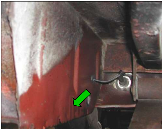
Trunk drop surface. No sealer at bottom edge
