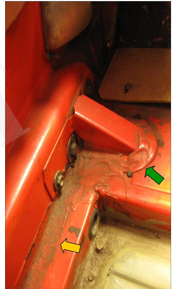
During periods of time in 65 production at San Jose the taillight panel to rear trunk floor seam sealant was applied much neater and did not require nor get, spread out with a rag as the one in the picture (yellow arrow) was. Instead a neat 1/2" bead is found.
