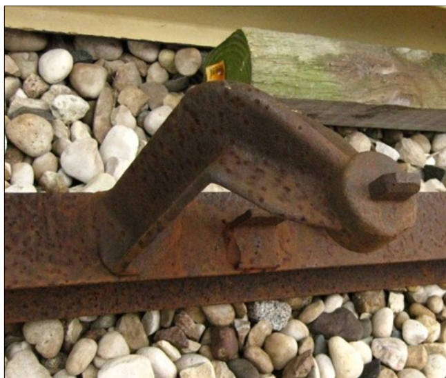
Here is a close up of the forward standard. At this point and one further back the cars simply sat on the stand with locator tab inserted in the cars frame rail.
